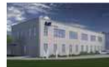
LS EV Poland./LSCP (Dzierzoniow) Automotive battery components Optical cable
